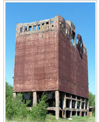
Ruins of the German synthetic petrol plant (Hydrierwerke Pölitz – Aktiengesellschaft) in Police, Poland
